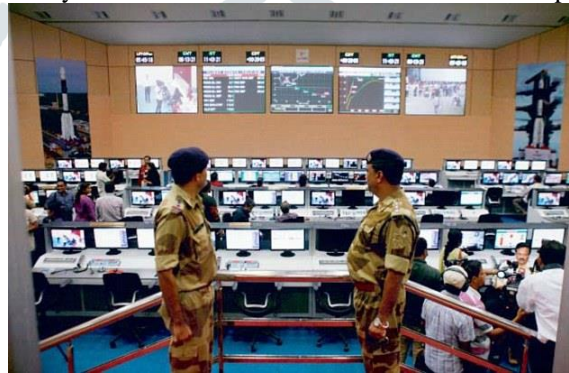
Fig. 3 Base unit or control room
