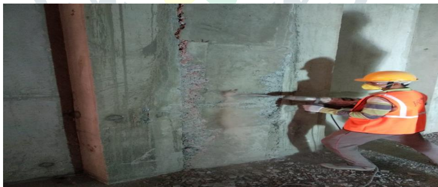
Figure 7.3 Rework of Column
