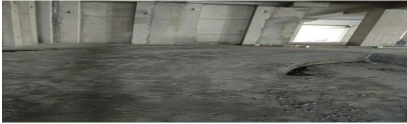
Figure 7.1: Ramp for basement
