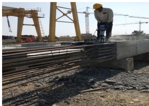
Figure 6.1.b: Column Breaking
