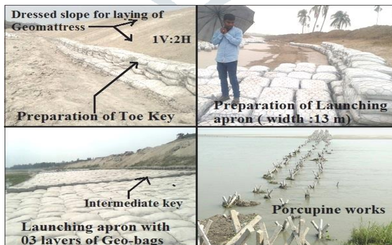
Fig. 9. Installation of geotextile bags and gabions at left bank
