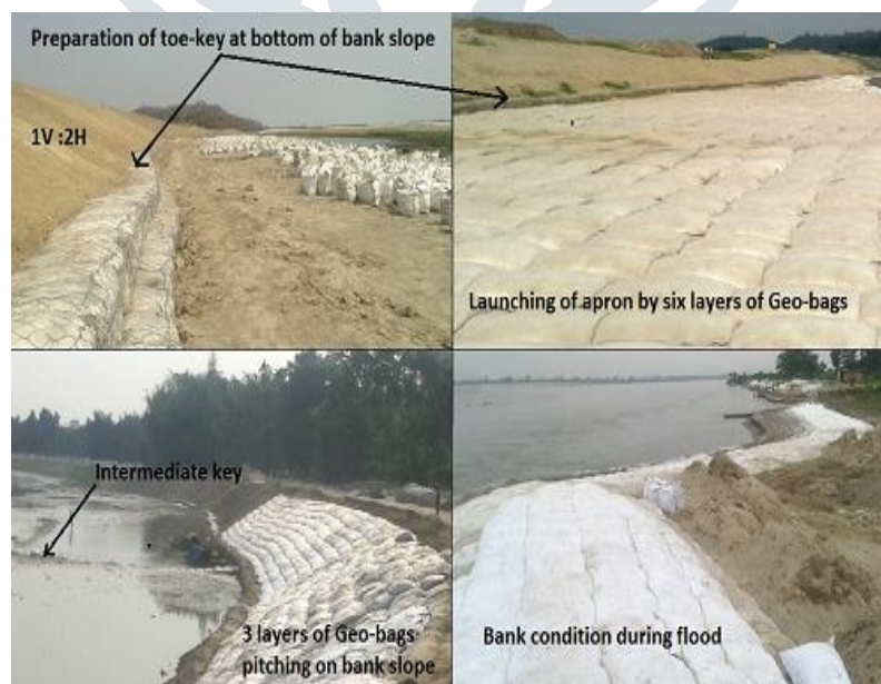
Fig. 7. Installation of Geosynthetics materials and Gabions at right bank
