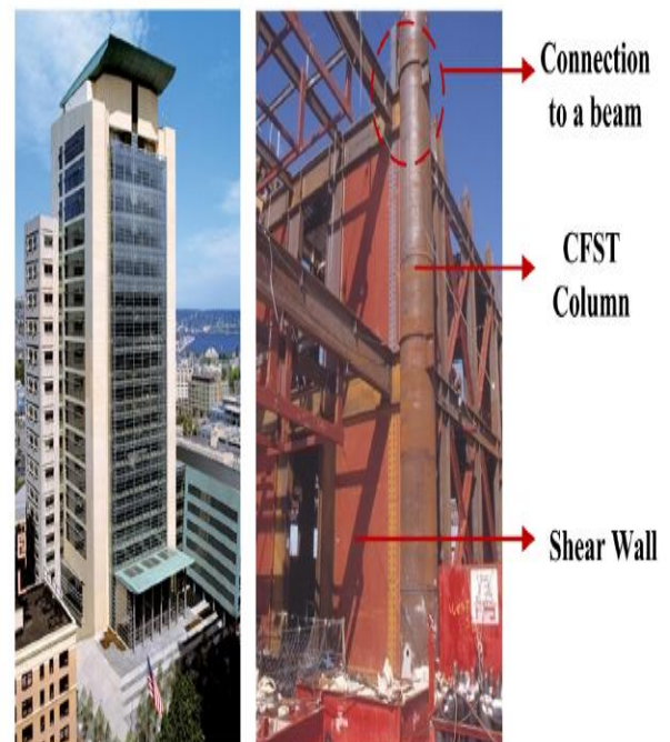
Fig. 1. Example of application of CFST member to a building column (U.S. Federal Courthouse, Seattle, WA, USA).
