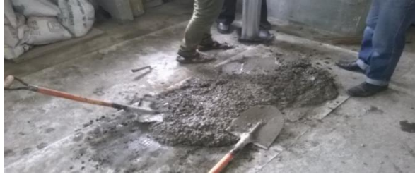
Figure 1 Preparation of concrete mix
