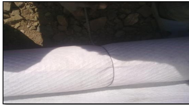
Figure 81: Perforated Pipe is hold by stitching with Binding Wire
