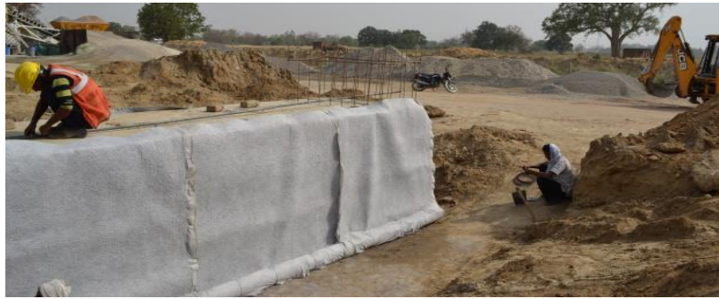
Figure 5: Cutting & Laying of Geo-composite Drain
