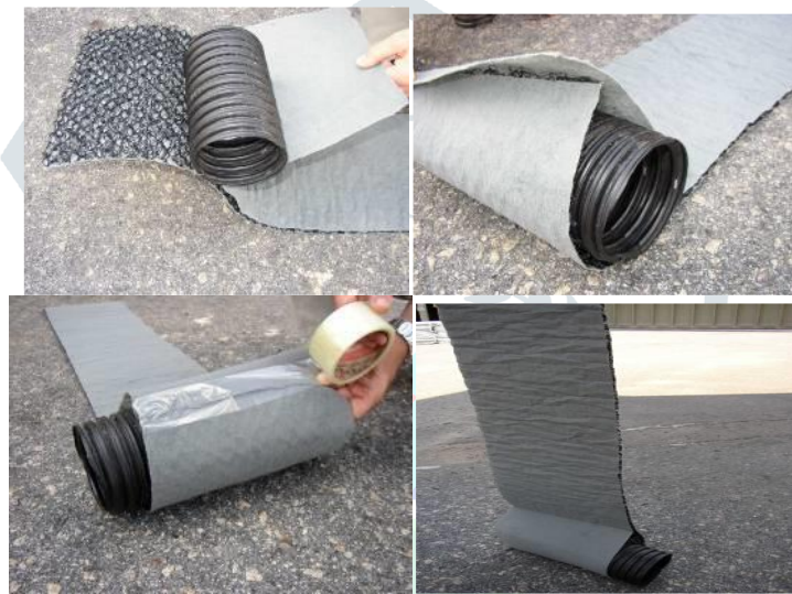
Figure 6: Sequence of fixing perforated pipe
