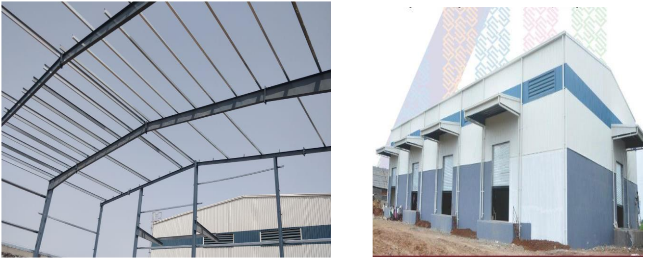
Fig 1. Structural frame and ware house
