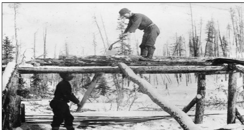
Fig-1: Traditional method of wood sawing.
