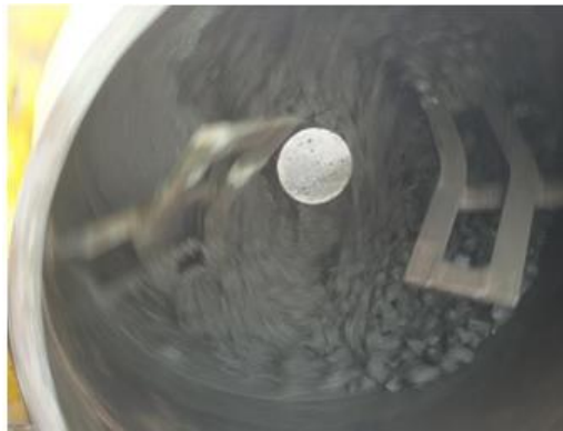
Fig 9: Mixing of Concrete
