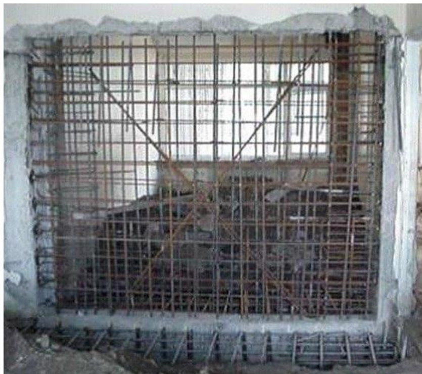
Fig 1.2. Additional Shear Wall
