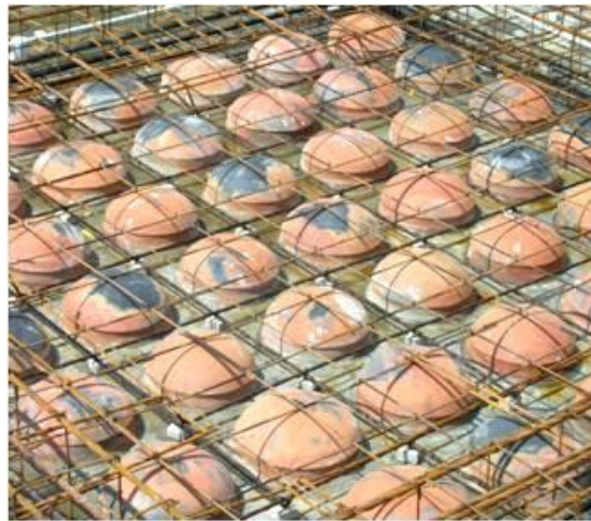
Figure 1 Clay pots used as filler material in the construction of filler slab
