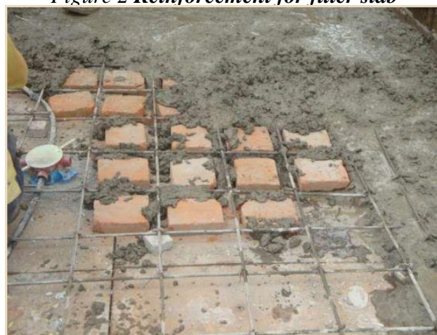
Figure 3 filling of filler material for filler slab
