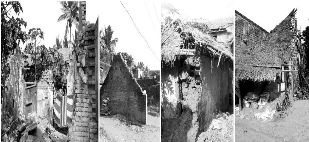
Figure 1 Damage of kutchha houses and semi-pukka houses of fishermen due to tropical cyclone, 2019, Somolo Island. Source: (Author).
