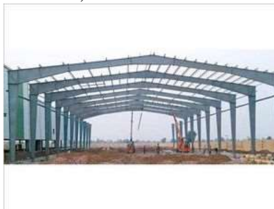
Fig .1: Example of PEB structure
