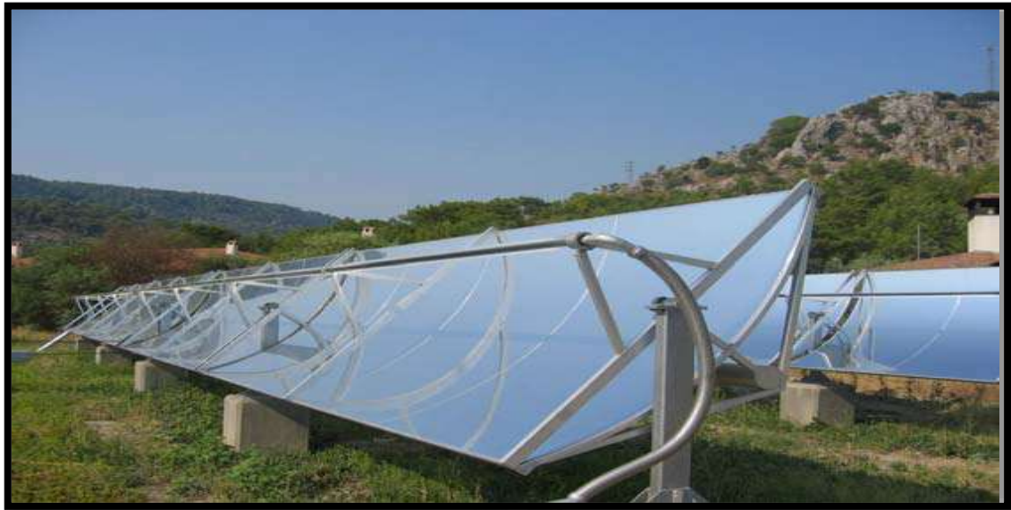
Figure-5 Alanod Polished Aluminium
