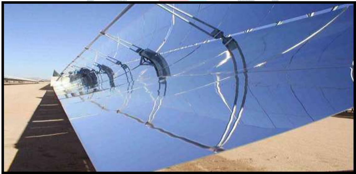
Figure-4 ReflecTech Silvered Film
