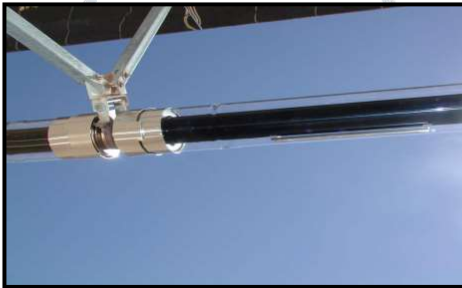
Figure 7- New Solel UVAC HCE New HCE
