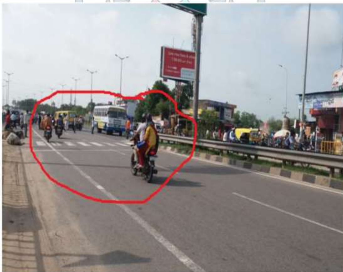
Fig 5 Unsignalized intersection and Zebra crossing faded away
