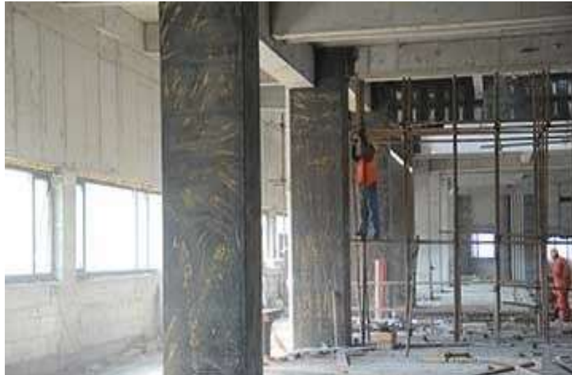
Figure 5.8 : Column strengthening
