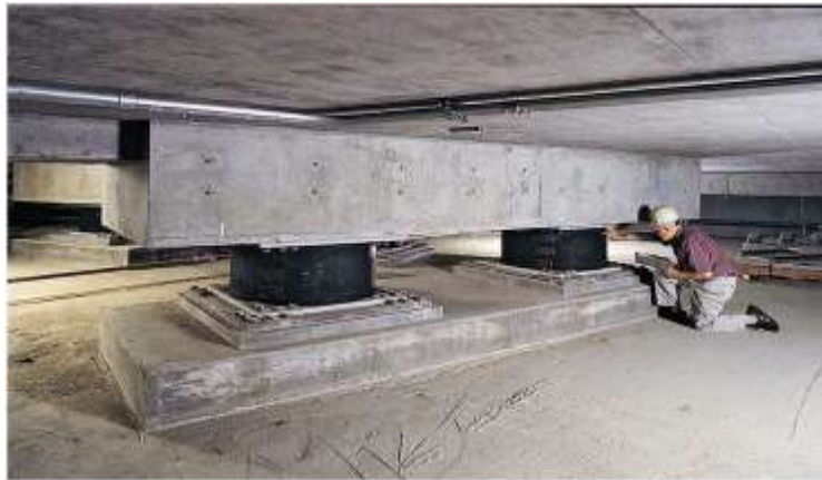
figure 1.1. base isolators [3]
