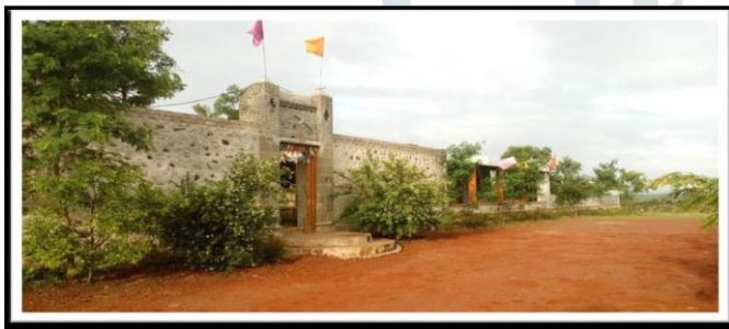
Figure 4.3 Entrance of the center
