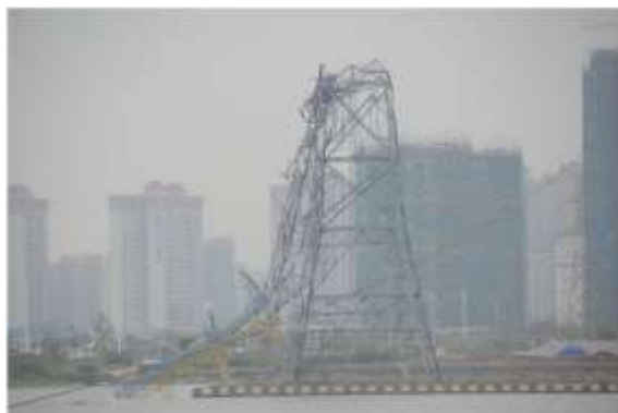
(a) collapse of tower N7
