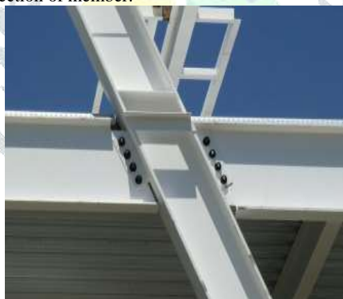
FIG 2: CONNECTION OF MEMBER
