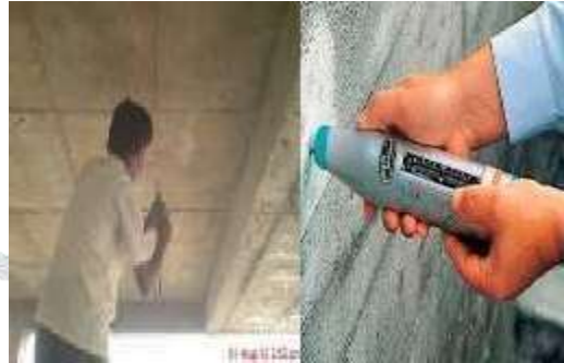
Fig 4: Non-Destructive Test [NDT] on Column and Slab in Building
