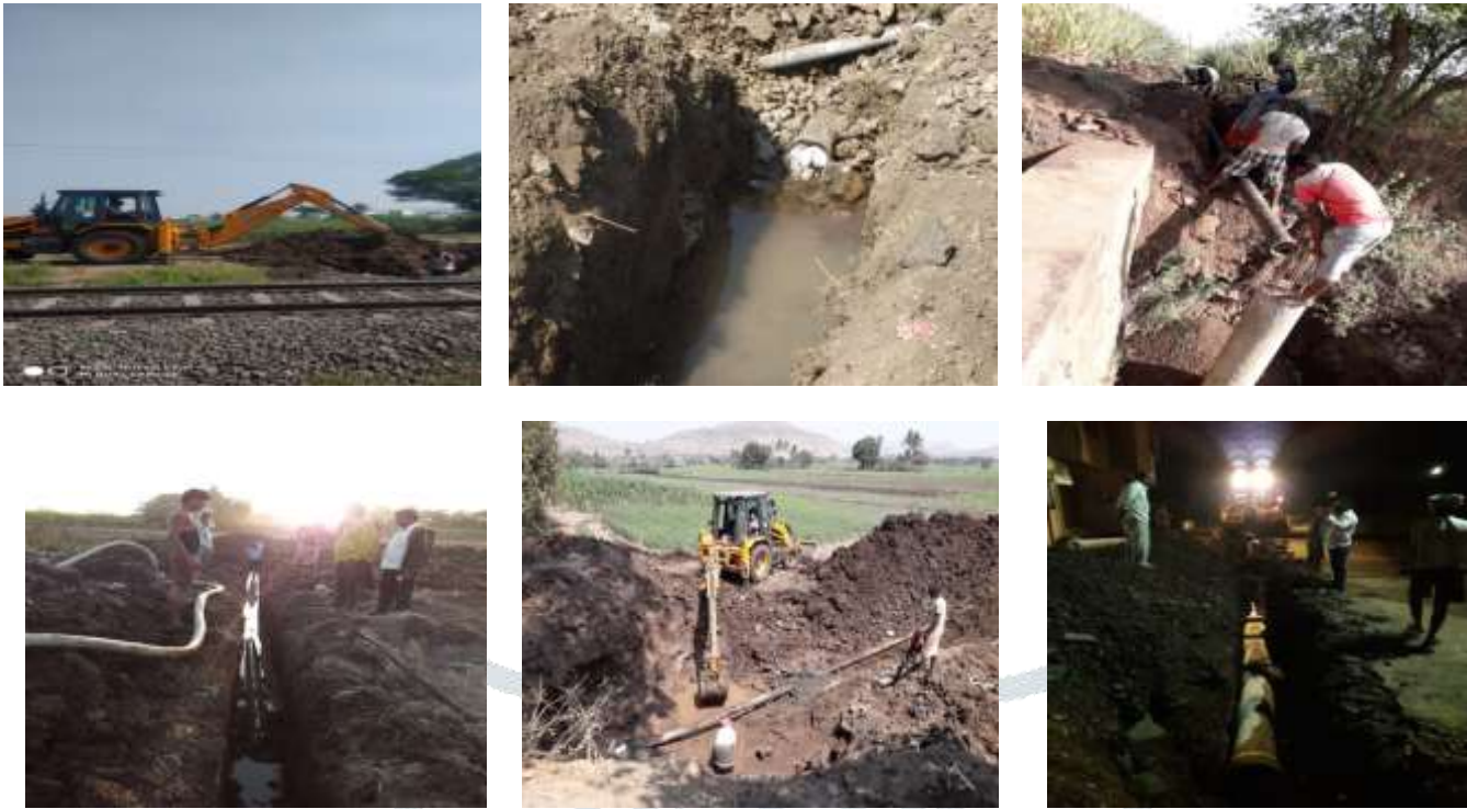
Figure 4.2 Actual photographs of site
