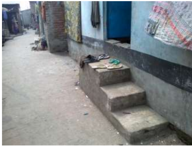
Figure-2: Wall to protect water of flood and water-logging at Dhaka Match Factory slum (Source: Author)
