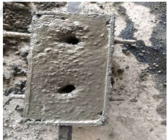
Figure: placing of concrete in mould for interlocking block.
