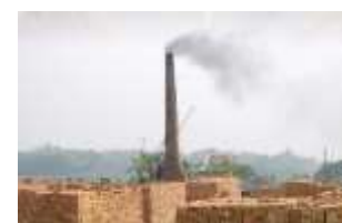
Figure 6 showing bricks Kiln
