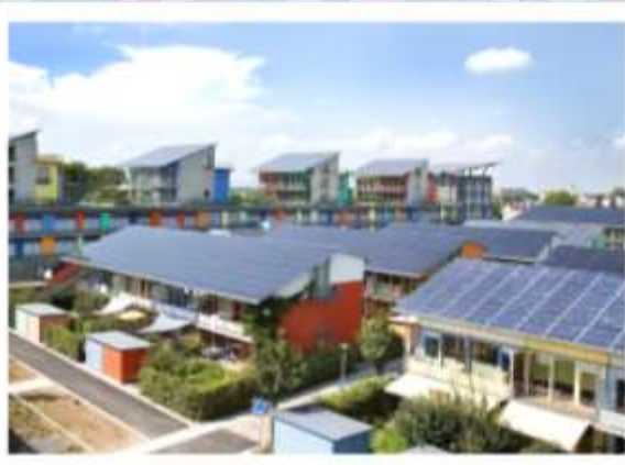
Fig no. 4.8 Photovoltaics
