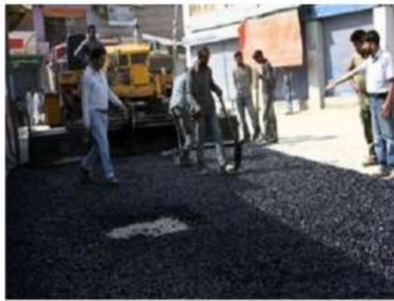
Fig. 1. Polymer Modified Bitumen at Srinagar National Highway
