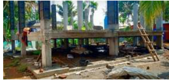
Figure 9 Pile dwelling under construction
