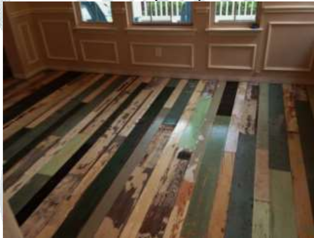
Flooring made up of Recycled wood.
