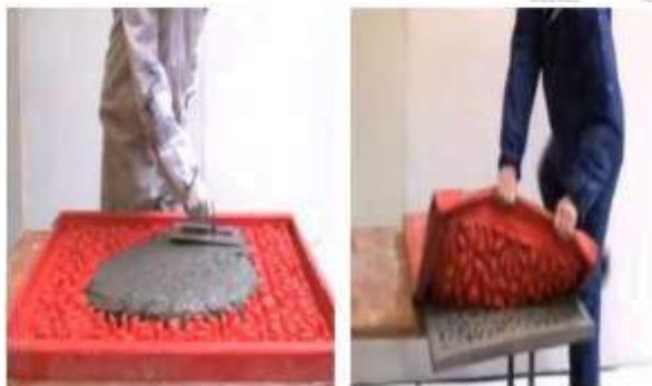
figure:- 2 pre-mixed and casting process
