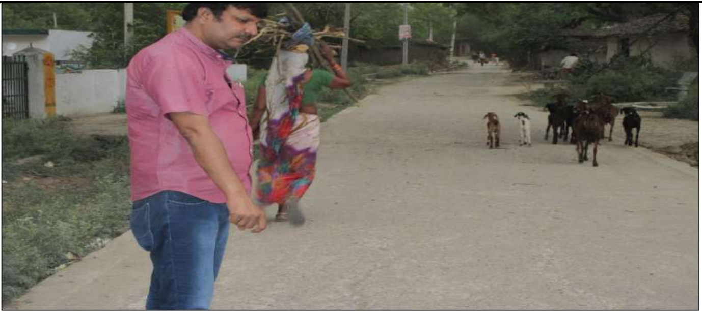
Sumerpur - Banki - Dharampur marg distt- Hamirpur (U.P.) cement concrete pavement in abadi portion
