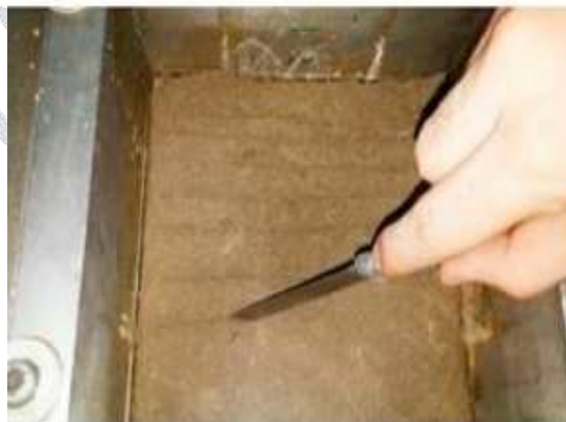
Fig.8 scratching the surface of each layer for proper bonding
