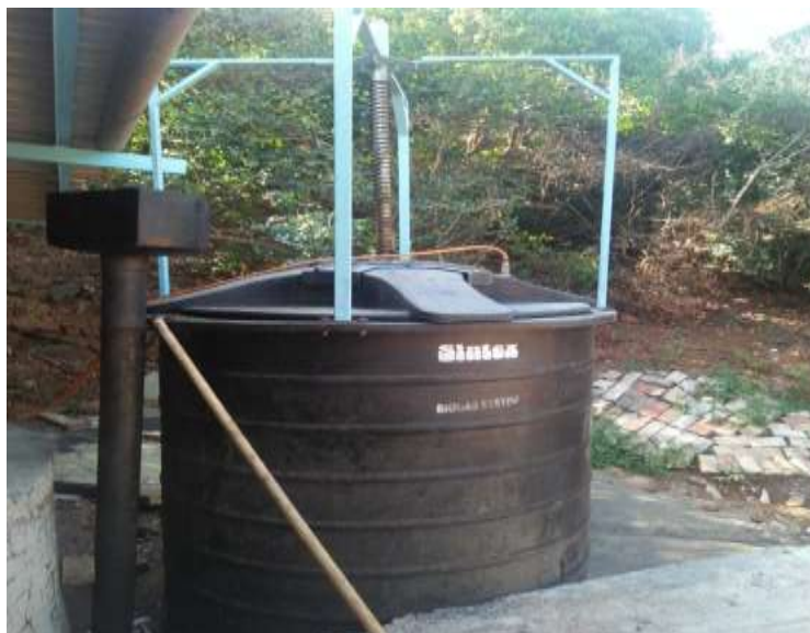
Figure1. Bio Gas Plant at Sairam Mahableshwar
