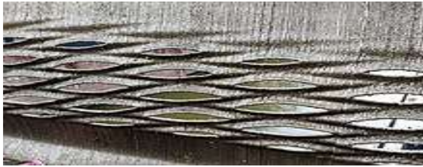
Fig. 4 Detail of the Stooftbrug in Amsterdam, the world's first 3D-printed metal bridge.
