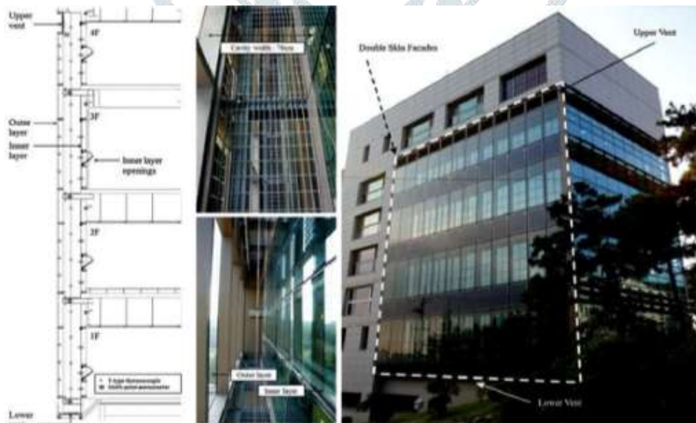
Fig (3): actual image of double skin photovoltaic facade
