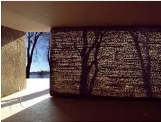
Fig 1 Translucent concrete wall
