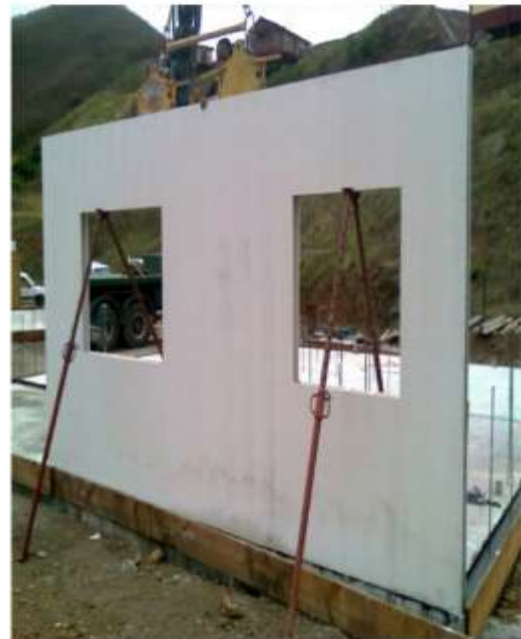
Fig. 13. Erection of GFRG panels over plinth beam at site.
