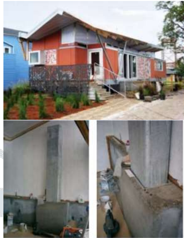
Figure 4 The FLOAT House, New Orleans. Elevation, interior guide post and sleeve details.
