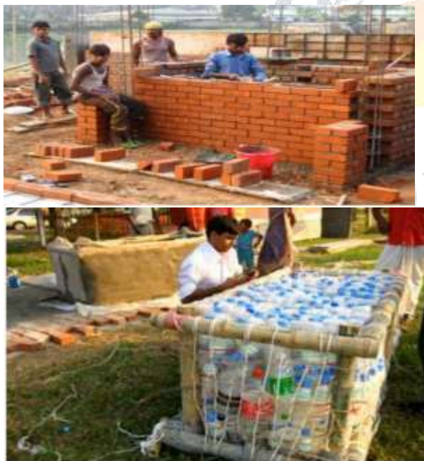
Figure 7 The LIFT House in Dhaka, Bangladesh. Concrete and brick base structure under construction; buoyancy block made of recapped, recycled plastic bottles.
