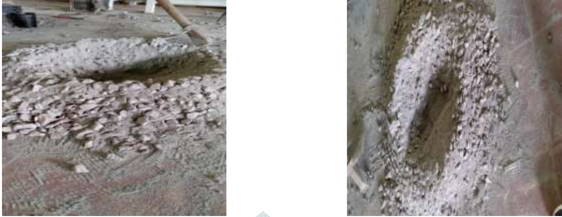
Fig. 1. Dry Mixing of fine aggregate, cement, coarse aggregate.
