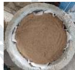
Fig. 7 Drainage layer of sand (at top)
