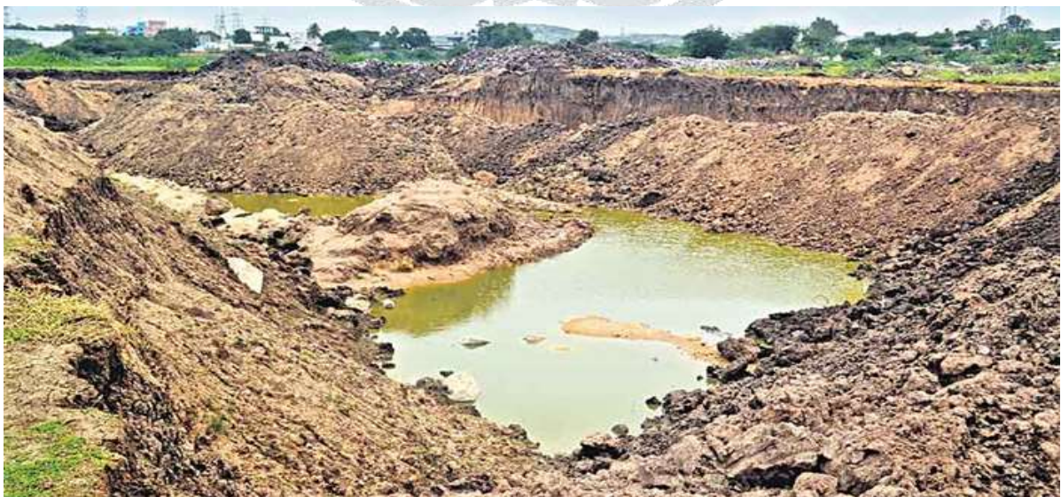
Fig. 2 Nala Dipping and Widening
