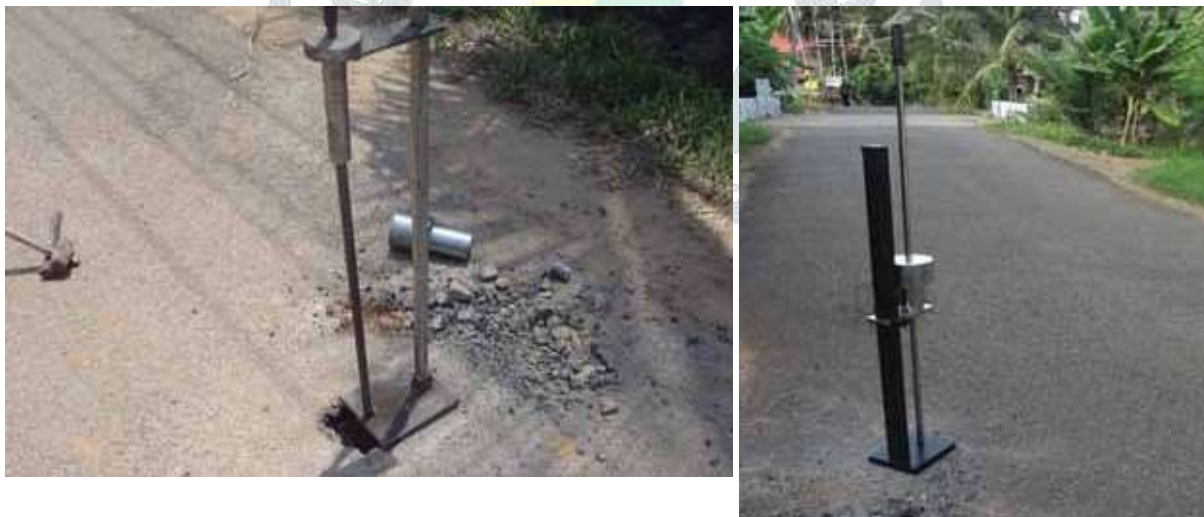
Fig: 5 Photograph of the DCP Test Setup
