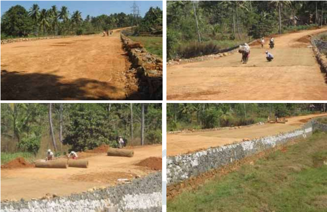
Fig:2 Construction of Coir geotextile Reinforced Pavement
