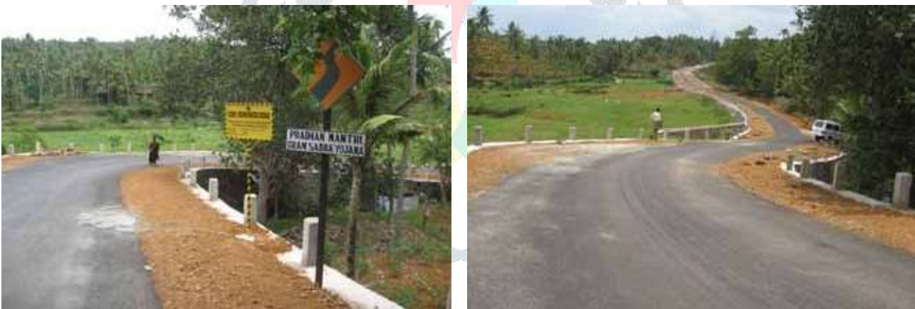
Fig:3 Photograph of the finished Coir Geotextile Reinforced Pavement
