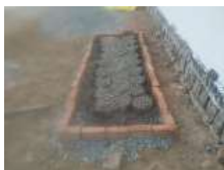
Fig 1 Placement of concrete and geo cell
