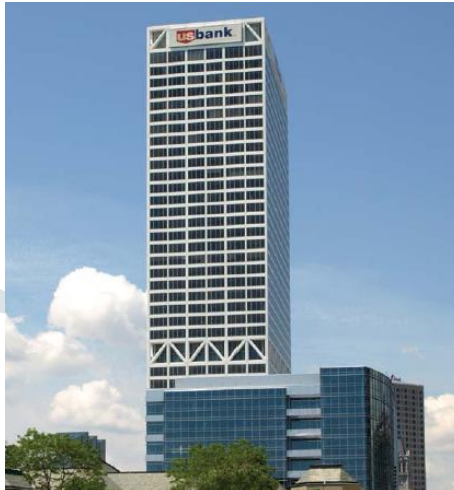
Fig. 3. U.S Bank Centre, Milwaukee, USA.
