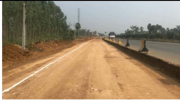
figure 1. soil subgrade.
