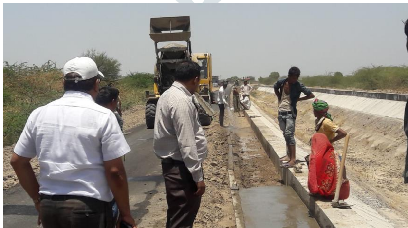
Figure 2 Construction of canal
