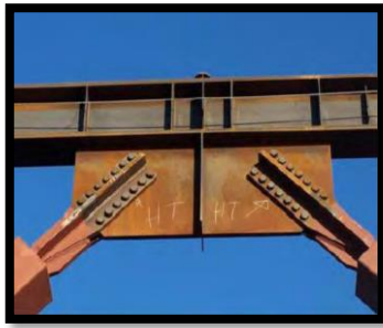
Figure 4 Bolted connection
