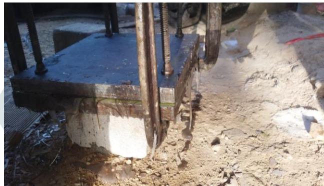
Fig.12. fabrication process step 5
