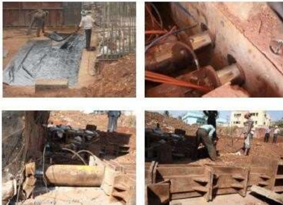
FIG-3: PUSHING BOX SEGMENTS USING HYDRAULIC JACK
