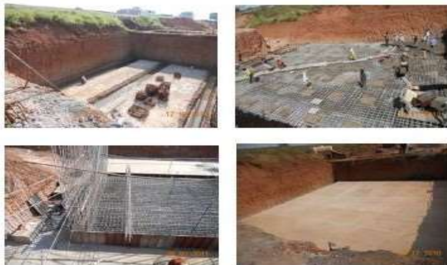
Fig-2 Construction of Thrust Bed
