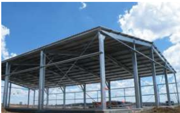
Figure 1: Pre-engineered building structure
