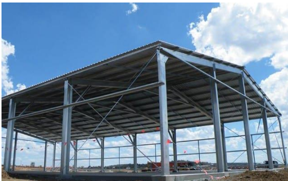
Figure 1: Pre-engineered building structure
